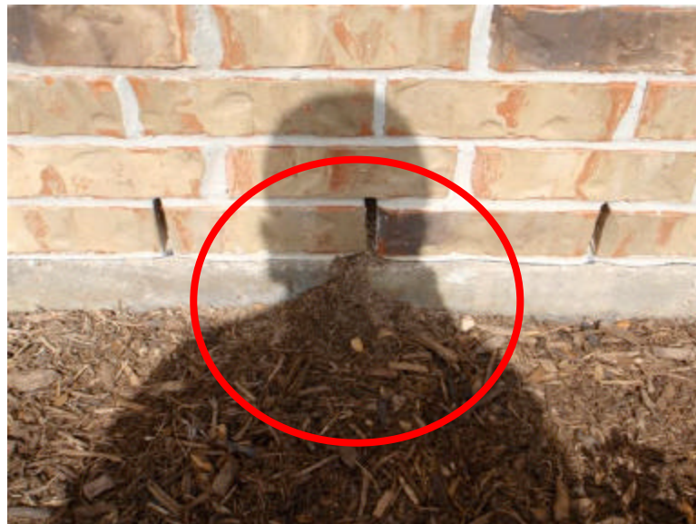
Ants entering house at brick weep holes, use insecticide treatment, do not seal up weep holes.
