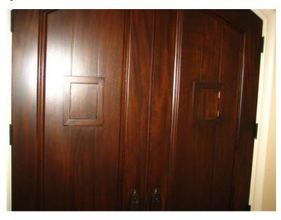
Recommend adding an interior lock/latch to small doors on front door. Doors can be pushed open from the outside to view interior of house.
