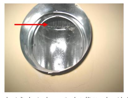
Recommend periodic cleaning dryer venting duct of lint to reduce risk of fire.
