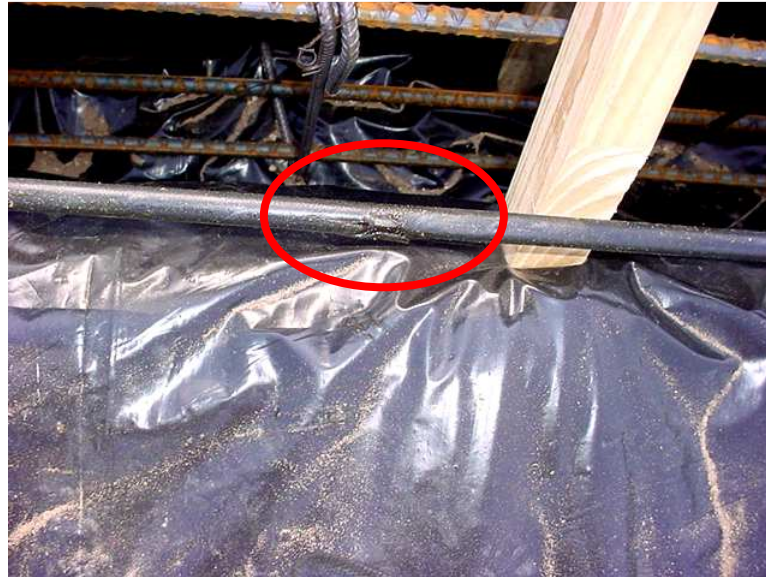
Observed tendons with nicks in sheathing not taped and greased.
